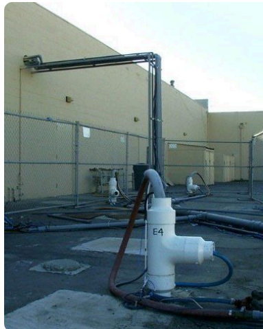
Vapor extraction and treatment, thermal and vapor extraction wellheads, and a HETR™ wellhead with burner and control enclosures.
