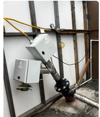
Vapor extraction and treatment, thermal and vapor extraction wellheads, and a HETR™ wellhead with burner and control enclosures.
