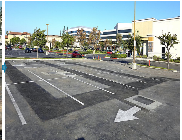
08 — Match existing surface conditions
