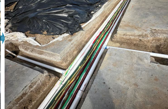
03 — Conduit & piping installed
