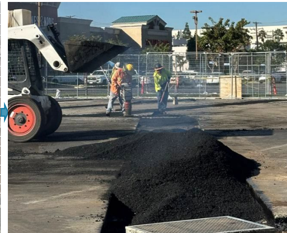
07 — Trench Backfill
