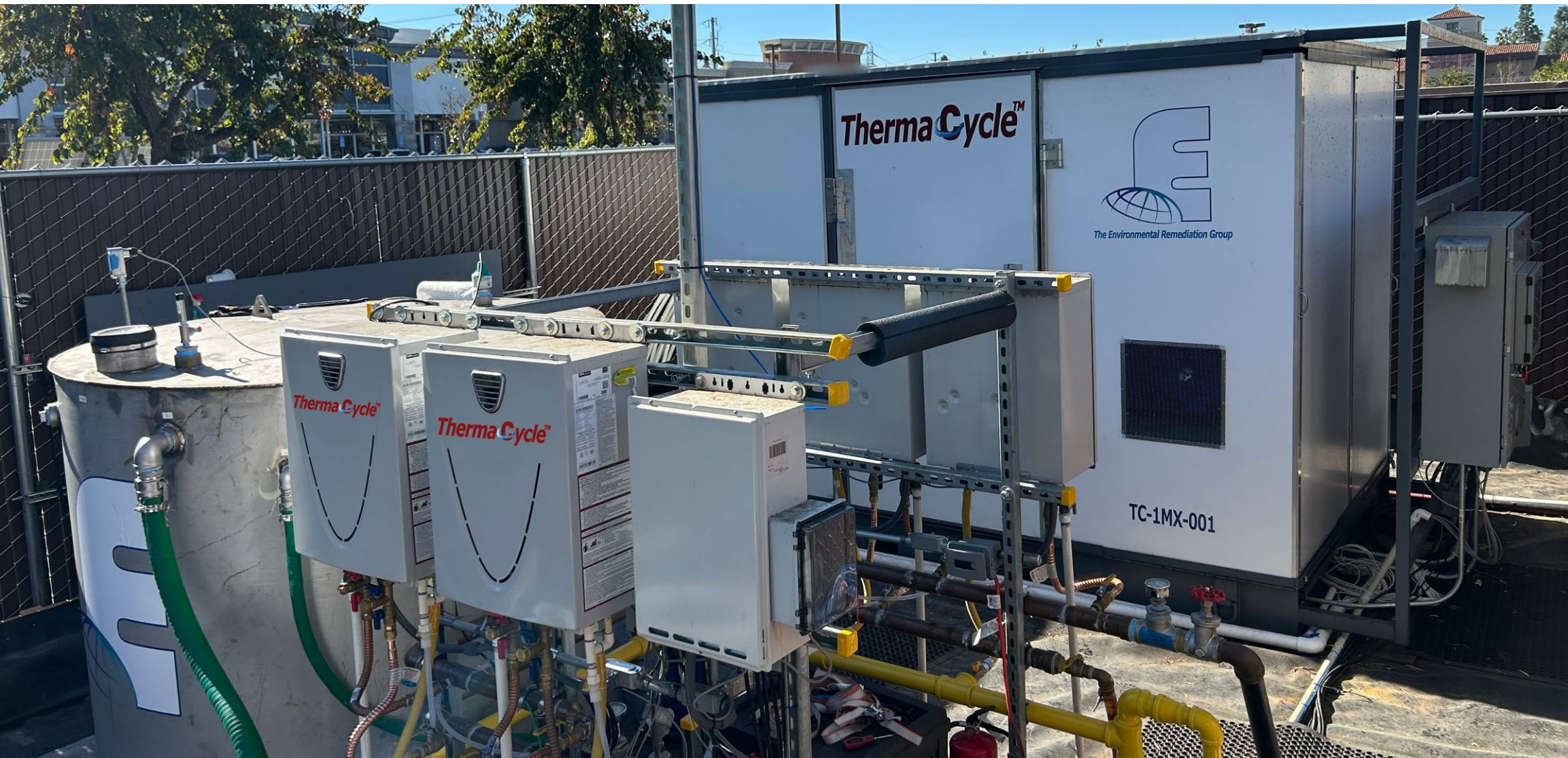
Internal Amendment Dosing Tank with mixer for soluble amendment injectate solutions (ie. water soluble nutrient amended carbohydrate blend).
